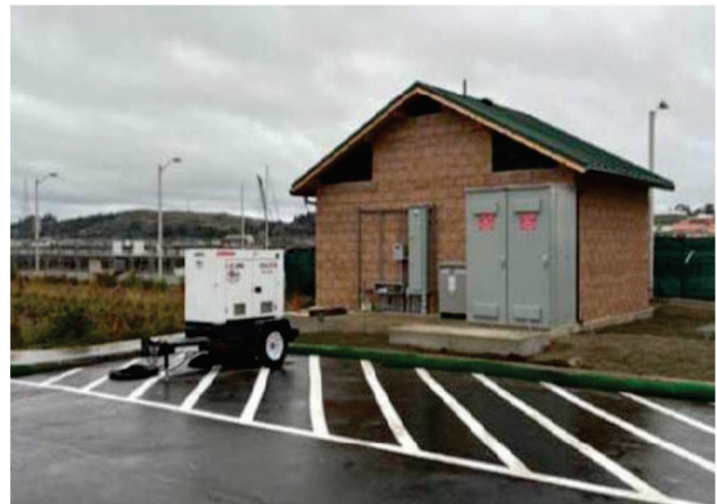
A new restroom building, landscaping and lighting were installed as part of the parking lot restoration.
