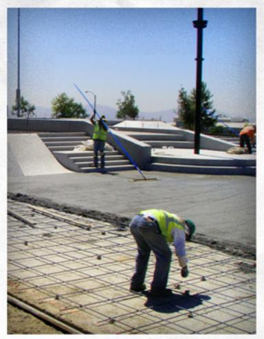
The final step in the "cap" method is the cap itself. The cap refers to the 4" of new concrete placed on top of the existing slab. This concrete receives a hard trowel finish and connects all of the skateable terrain built in step 1. After saw cuts and caulking, the park is ready to skate!
