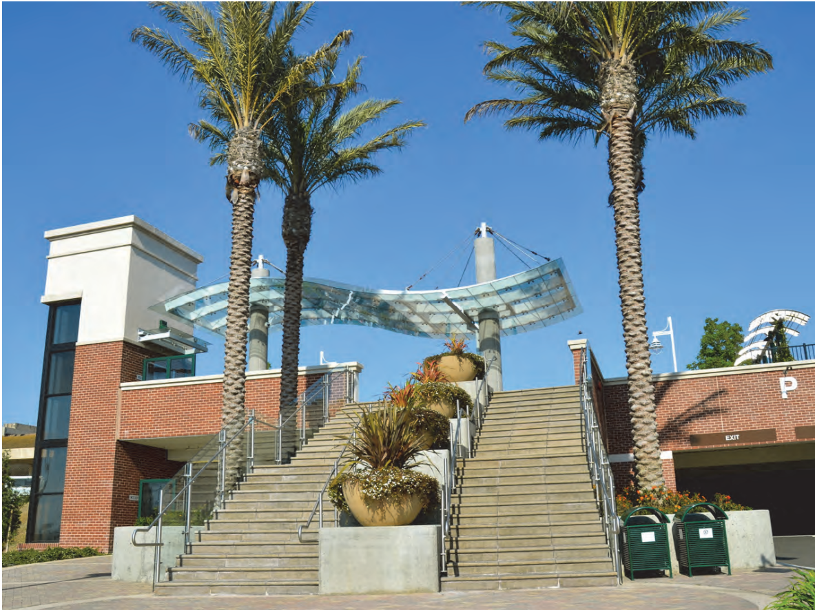
Vallejo Station Parking Structure
